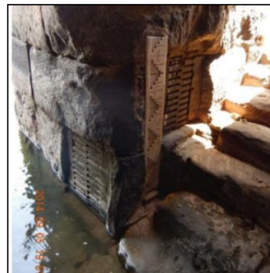
Fig.5 The Nilometer at Elephantine Island, consisting of Stairs and gauges.
