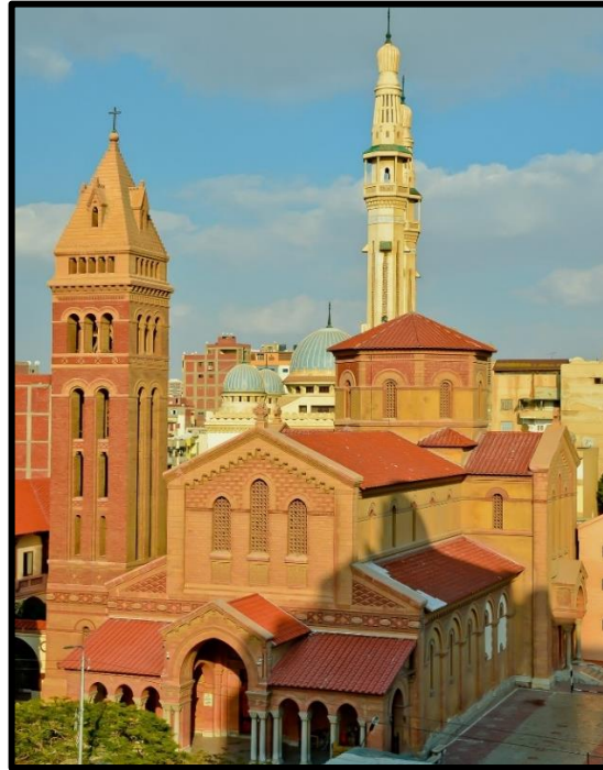
Pl. 6: Tower of Saint Mark Church (the French Church) in Ismailia. (By the Researcher)
