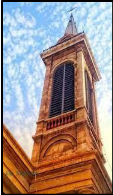
Pl. 9: Tower of Saint Eugenie Church in Port Said. (By the Researcher)
