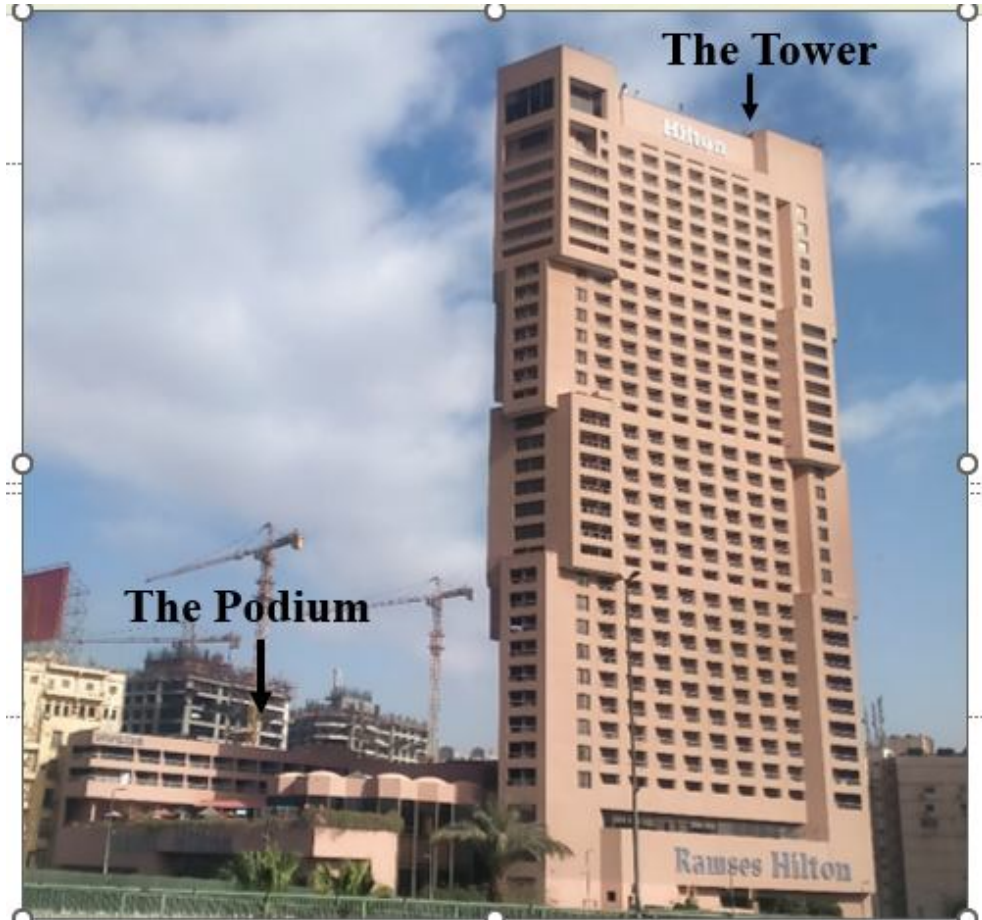
Fig. 5: The triangular tower and the podium of Ramses Hilton. Photographed by the author.
