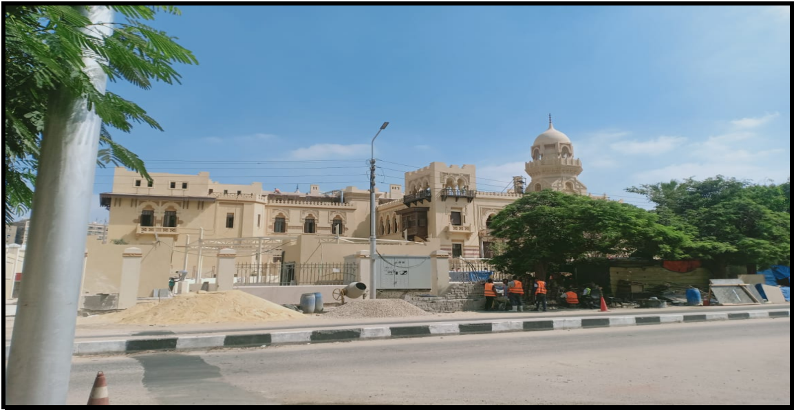
Source: The current restoration of Malak Jeshem Palace – the Researcher 2021.
