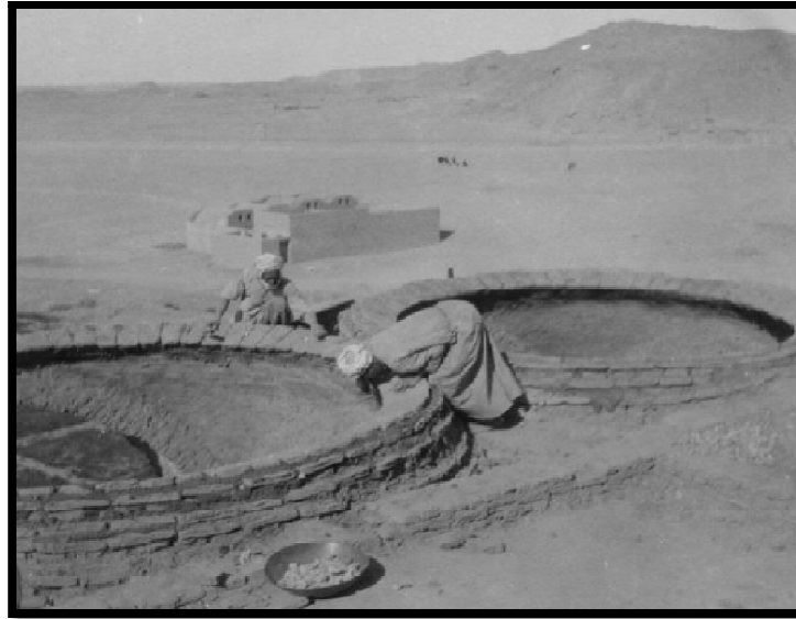
Figure 8: Clarke's house in Elkab, showing the construction of two domes above the entrance arcade (Photograph by Clarke, circa 1906). Courtesy Griffith Institute. University of Oxford, Somers Clarke Mss. 19.40.06.
