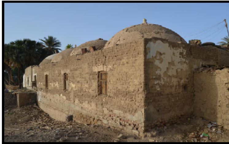
Figure 6: Four domes constructed from mud-brick within the workers' houses at the Edfu Railway Station, designed and executed by architect Somers Clarke, and still standing to this day. Photograph by the researchers.
