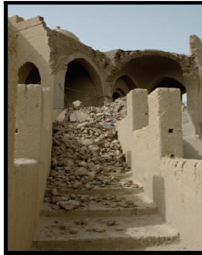
Figure 14: View of the eastern side of the arcade, 2009 after the collapse, after Nicholas Warner, Saving Bayt Clarke: a mud brick masterpiece by the Nile , fig. 10.
